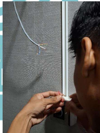
Instalasi push button fingerprint
