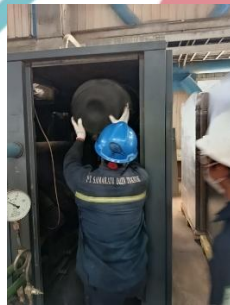
Gambar 3 Cleaning Filter Udara
