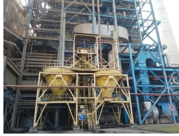
Gambar 9 Bottom Ash Silo
