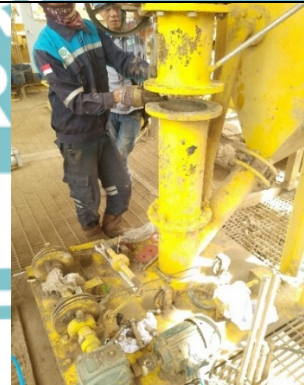
Gambar 5.6 Penggantian Knife Valve FAS B
