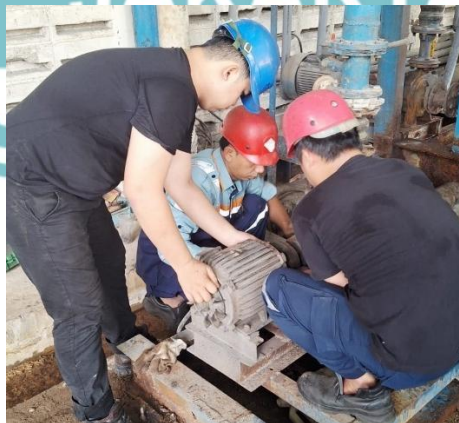
Gambar 8 Assembly Pompa Cooling Tower
