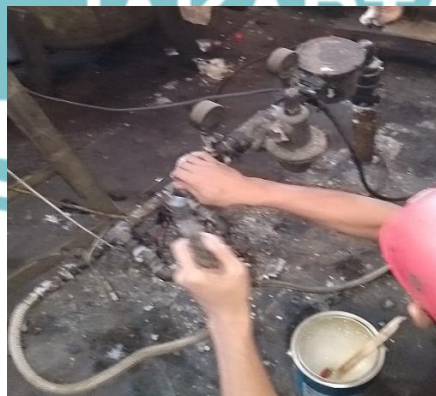
Gambar 5 Pemeriksaan Kebocoran Pipa Gas Plant Casting
