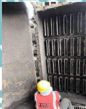
Gambar 1.3 Proses penggantian bag cloth bag filter (482-BF1)
