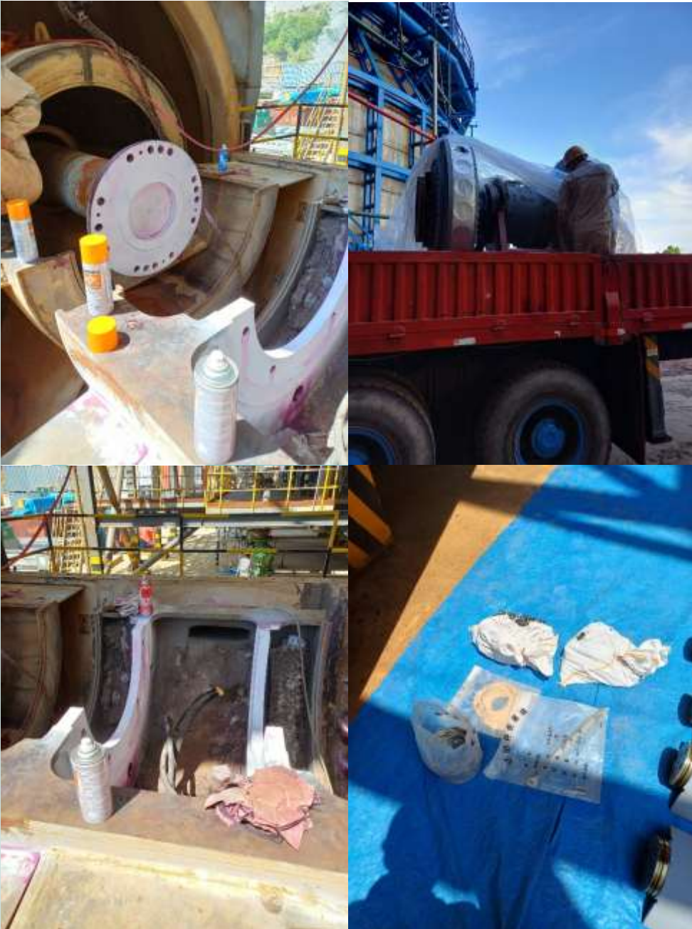
Lampiran 4 perbaikan induced draft fan
