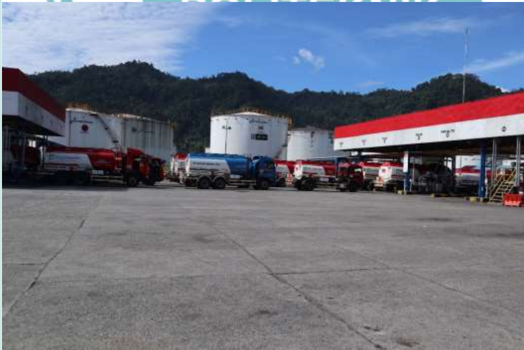
Lampiran 2 – Area filling shed PT Pertamina Patra Niaga IT Teluk Kabung
