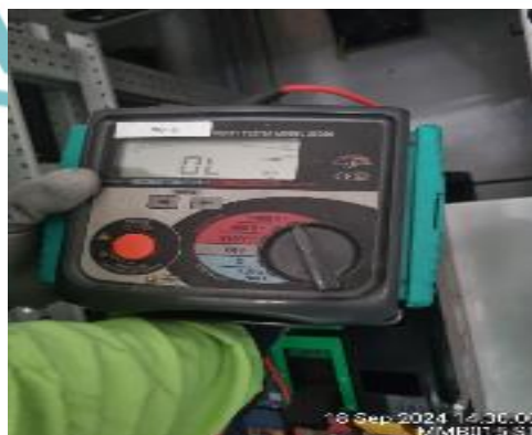
Gambar 4. 10 Insulation Test (Megger)
