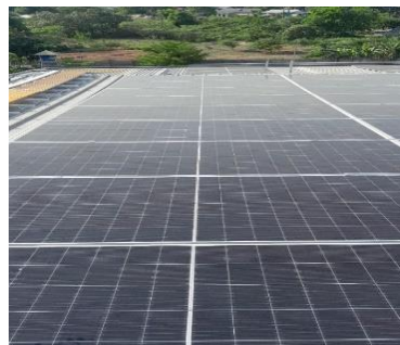
Gambar 4. 3 panel surya Monokristalin
