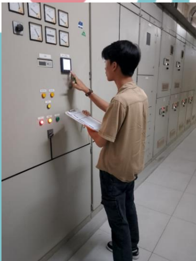
Lampiran 5 Pengecekan Cooling Tower
