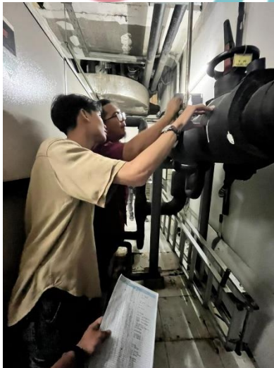
Lampiran 3 Pengecekan Motorize Valve
