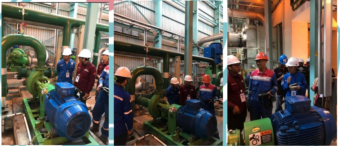
18. Running Operation Test ACWP dan CCWP Unit 4
