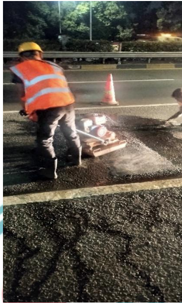
Gambar 3. 13 Patching Aspal
