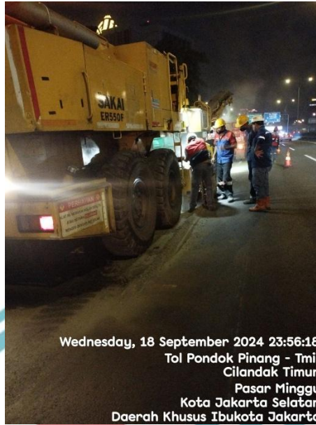
Gambar 3. 15 Scrapping, Filling, & Overlay
