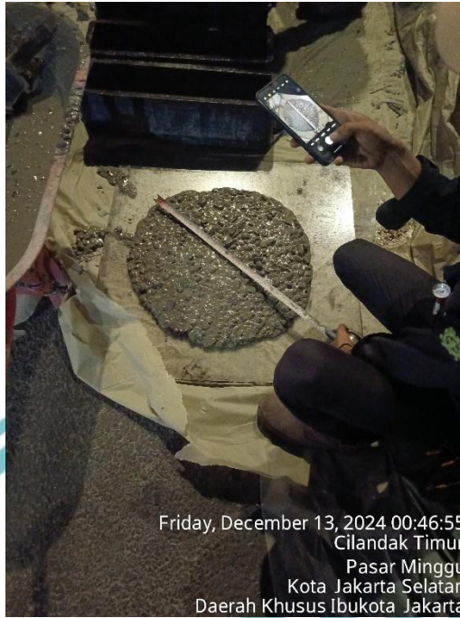
Gambar 3. 63 Uji Slump Readymix
