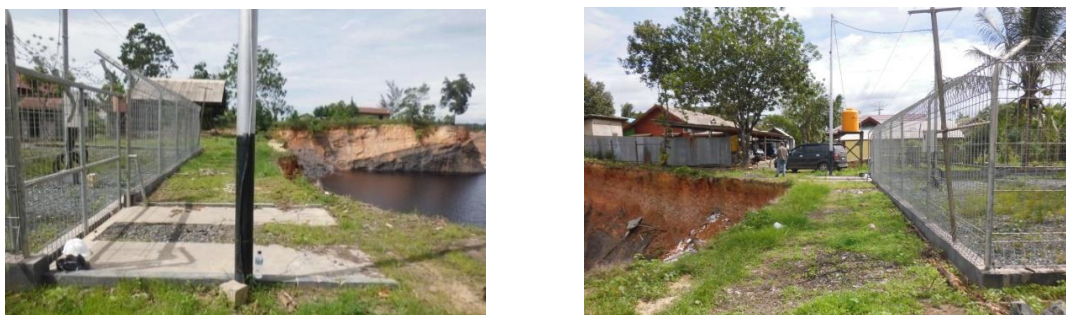
Figure 4. Pathway and edge of the fence after eroded
