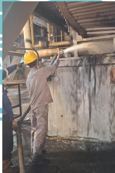
Cleaning MSM Unit 1
