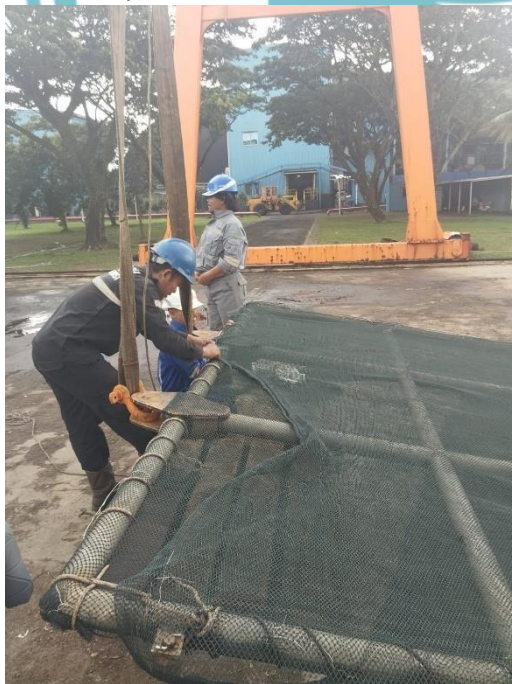
Pemasangan Temporary Screen TBS
