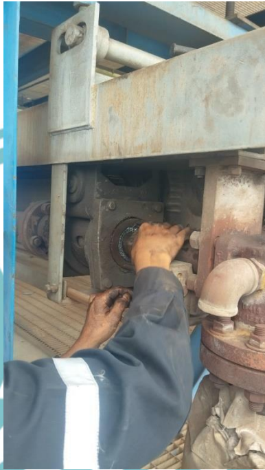
Penggantian Gland Packing L10 #1
