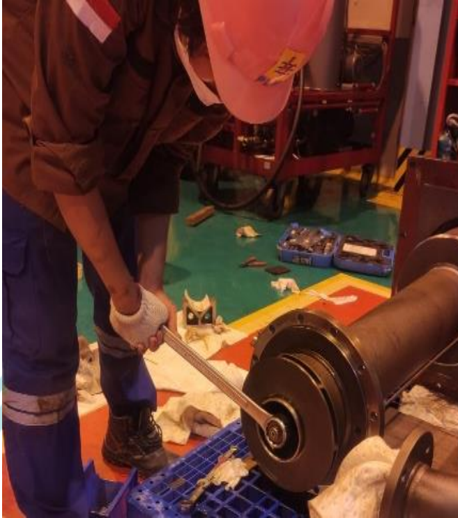
Lampiran 3 Dokumentasi kegiatan Penggantian Bearing main lube oil Pump
