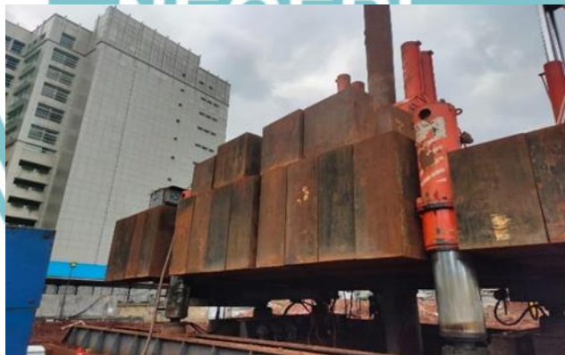
Gambar 3. 41 Hydraulic State Pile Driver Sumber : Dokumen Pribadi
