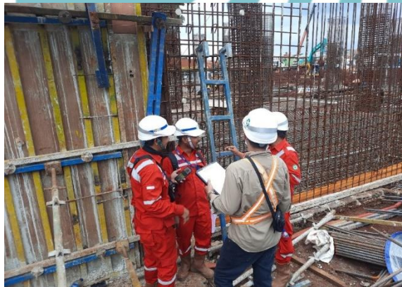
Gambar 3. 23 Checklist Penulangan Retaining Wall
