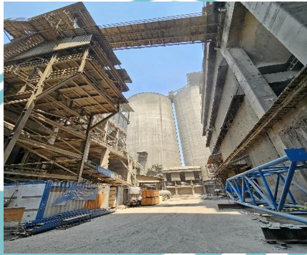
Gambar 2.4 Plant 3-4 PT Indocement Tunggal Prakarsa Tbk
