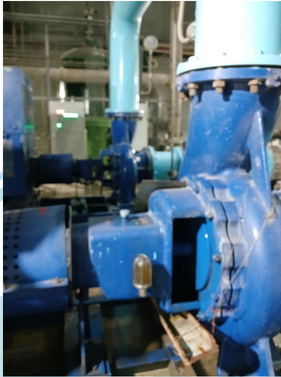
Gambar 3.3 Close Cycle Cooling Water Pump
