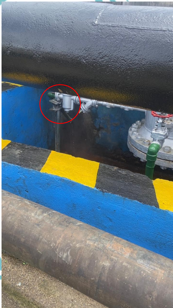
Gambar 2.2 condensate drain pot
