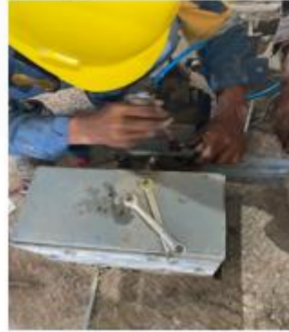
Install pneumatic actuator
