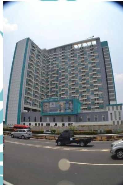
Gedung H Residence MT Haryono
