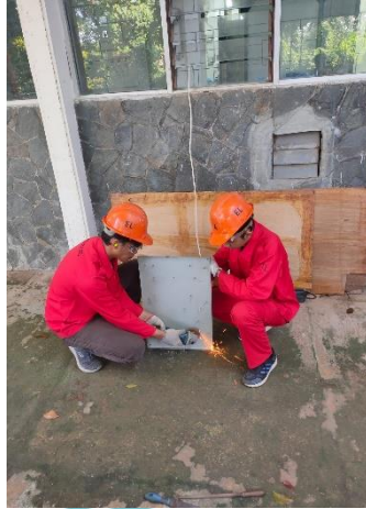
Lampiran 5 Proses Gerinda Baut Base Plate Panel
