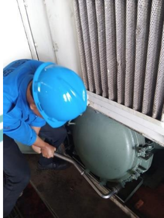
→ Proses membuka baut housing filter oli engine.
