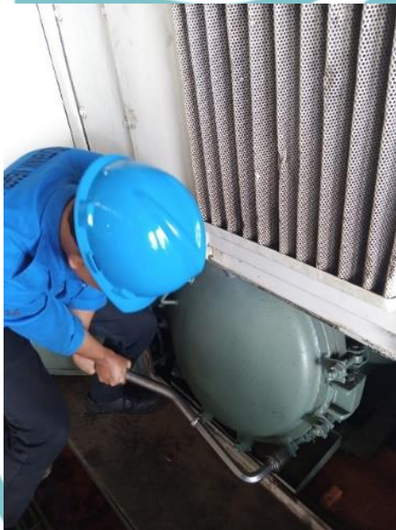
Proses pembukaan housing filter
