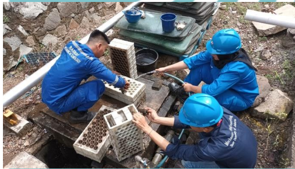
Proses pencucian filter udara
