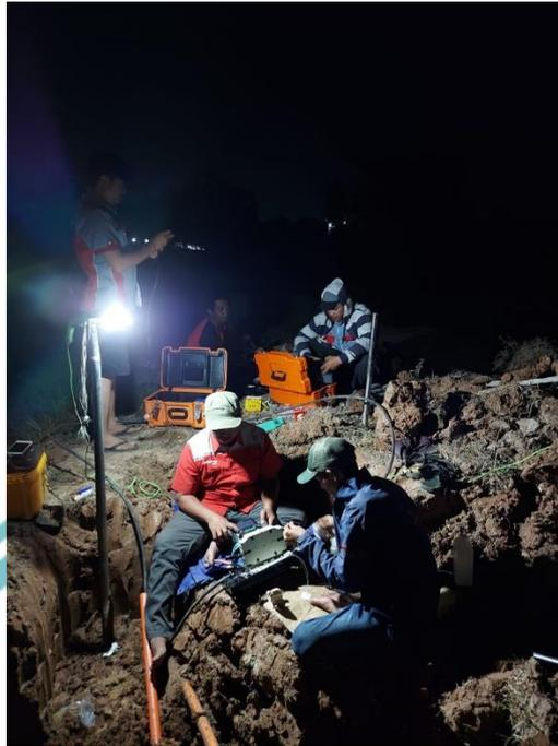
Gambar 3. 19 Proses Pelilitan Kabel di *Joint Closure*
